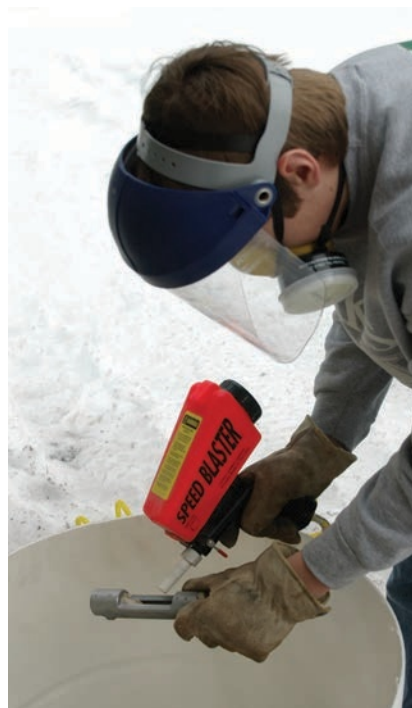
When sandblasting to rough-up parts, wearing face protection and a respirator is always essential.
